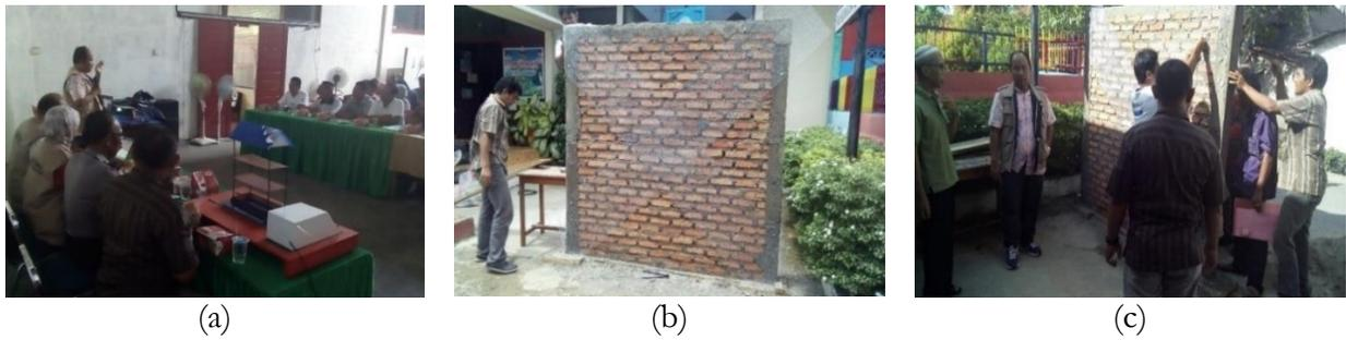
Figure 8. Community activities (a) Presentation of the material (b) Simulation of retrofitting a 2m x 2m wall using a 2cm x 2cm wire mesh and (c) Direct practice of making wall reinforcement.
